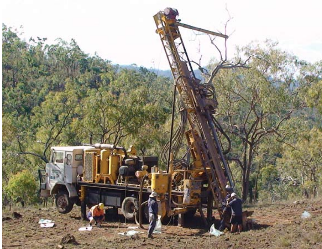
Drilling at the Gillian project
